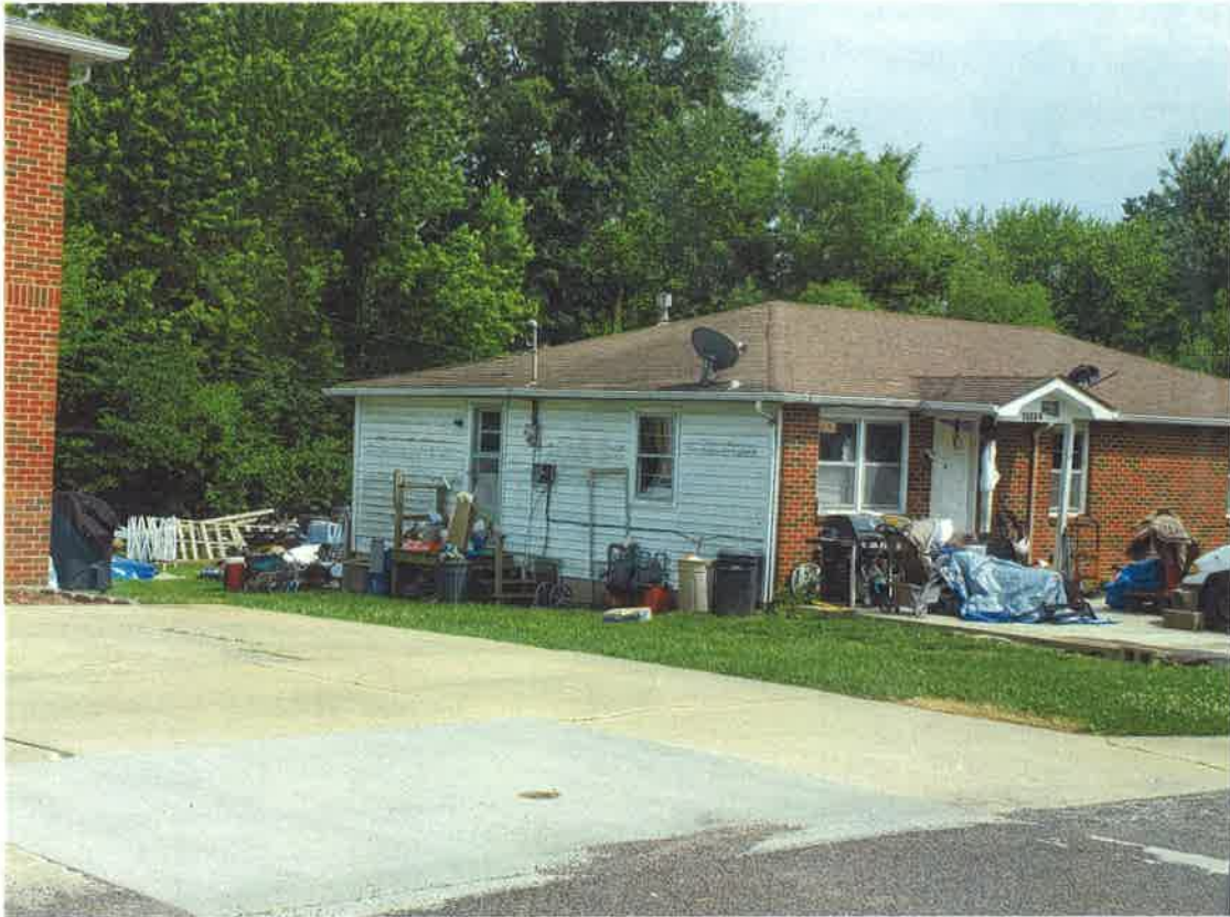
Photographs taken 6/8/20 @ ~ 3:30 pm 6008 N. Kent Drive A+B
