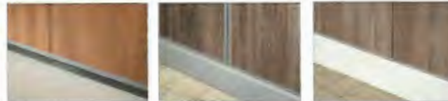
2" Reveal Base creates a subtle recessed transition to the floor
