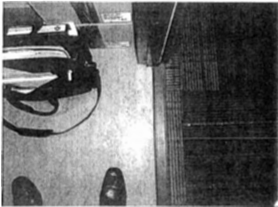
Image of flooring
