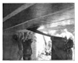
Installation of the CFRP Sheets
