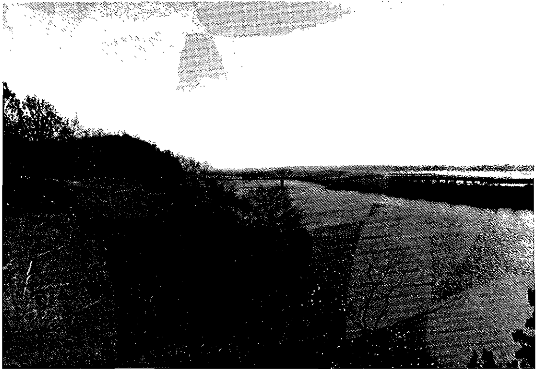
Photo 1 - Interstate Highway 70 spans the Missouri River downstream from Rocheport.
